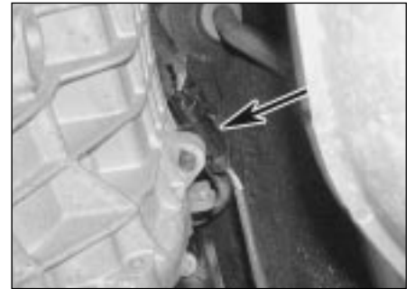
18.6 The oxygen sensor wiring connector (arrowed) is clipped to the side of the transmission unit
